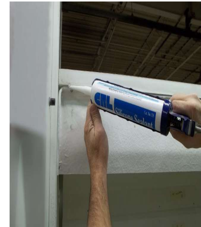
Caulk the interior perimeter of the Ceiling Panel joints with provided 100% silicone caulk.
