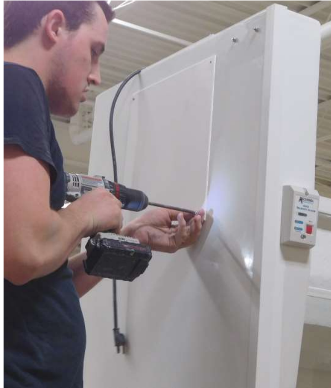
Install access panel over weight access area.
