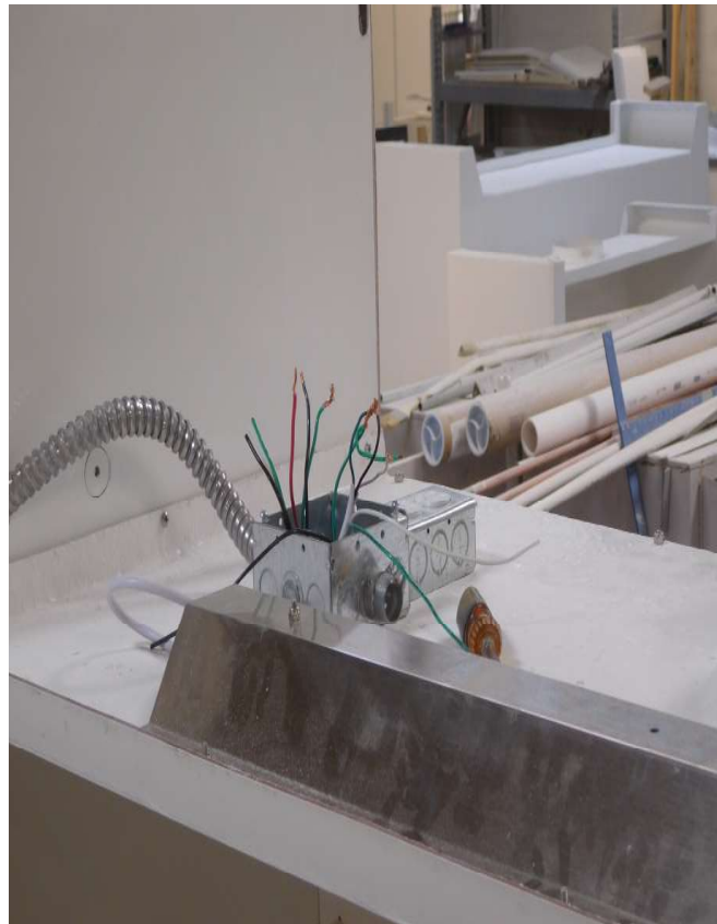
Have a qualified electrician hook up the electrical.
