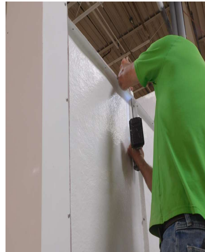
Secure Ceiling Panel to Side Shells with provided #8 or #10 sheet metal screws.
