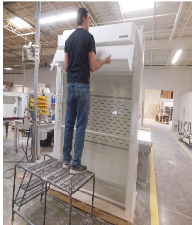
Install Front Access Panel.
